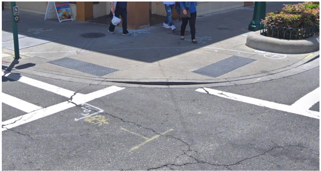
Figure 20: Directional Curb Ramps at the Intersection of Park Street and Santa Clara Avenue
