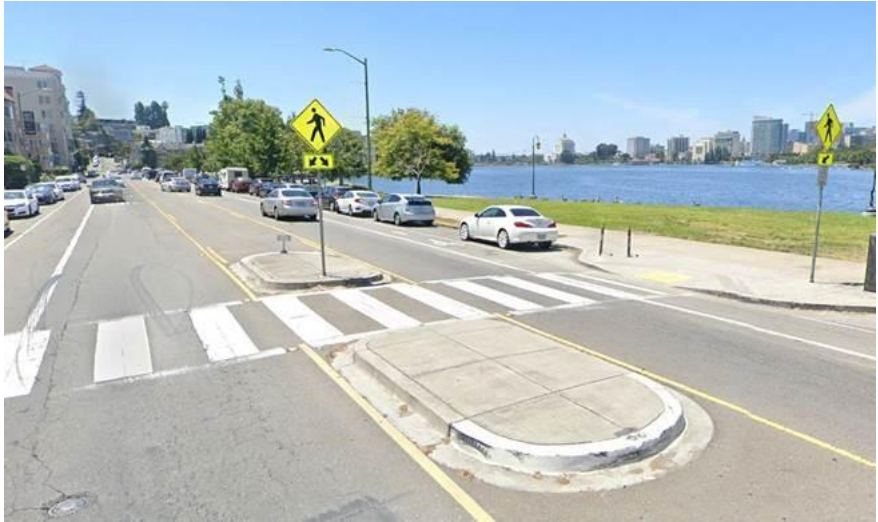
Figure 17: Median Refuge Island at the Intersection of Lakeshore Avenue and Cleveland Cascade in Oakland.
