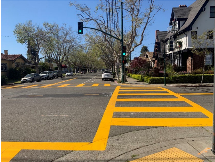
High-visibility crosswalks on Central Avenue
